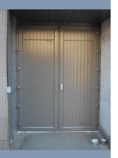
StormMeister was commissioned to provide an appropriate product to satisfy specific requirements, where the flood door not only to have to resist floodwater as the floodwater level rises but also as the floodwater level falls.
